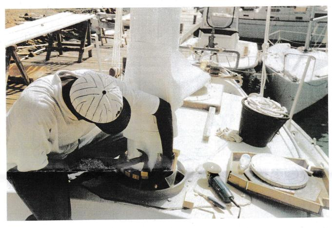
Having calculated the mast positions – with Mr v L's help again – Sandy glassed in substantial floors in the fo'c's'le and saloon, onto which Glen's fabricated mast steps were bolted.
