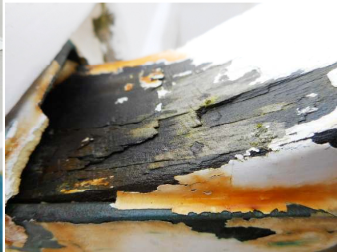
Fig 39 (below). Dampness in tiller by hood bracket.
