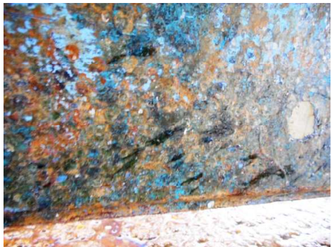
Fig 8. Detail of bottom of keel, showing evidence of minor worm / gribble damage.
