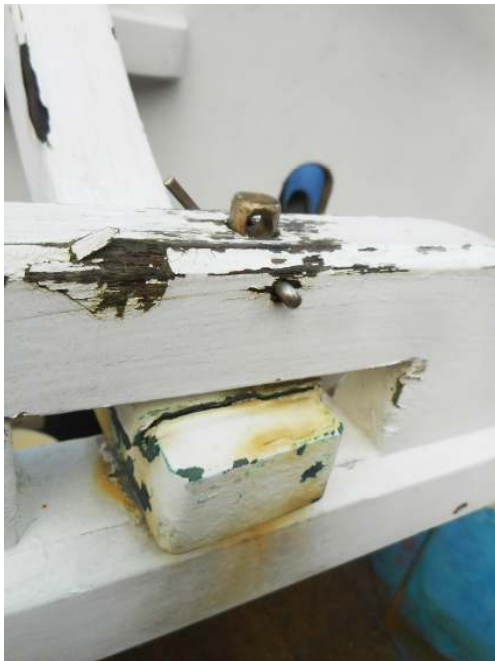
Fig 38 (left). Centre of crossbar, showing damp timber by hood bracket.
