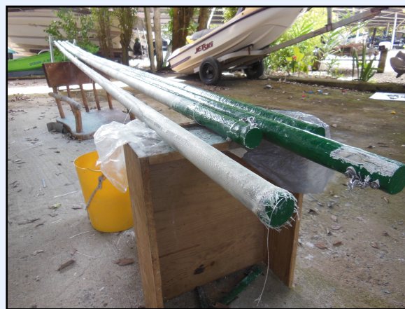
Repairing battens, Rio Dulce, August 2014
