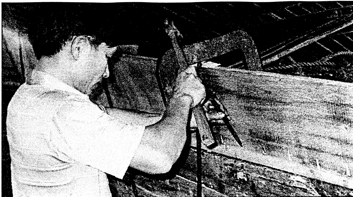
Figure 31 (above). The builder next drives home the nails using a long, triangular shaped nail set, until the nail ends just disappear into the wood of the triangular notch.
