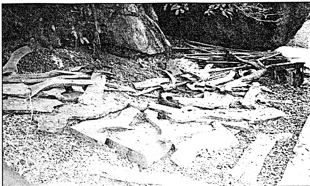
Figure 38. Curved, Grown Timbers at Tanzhou Air-drying in preparation for their use as frames.
