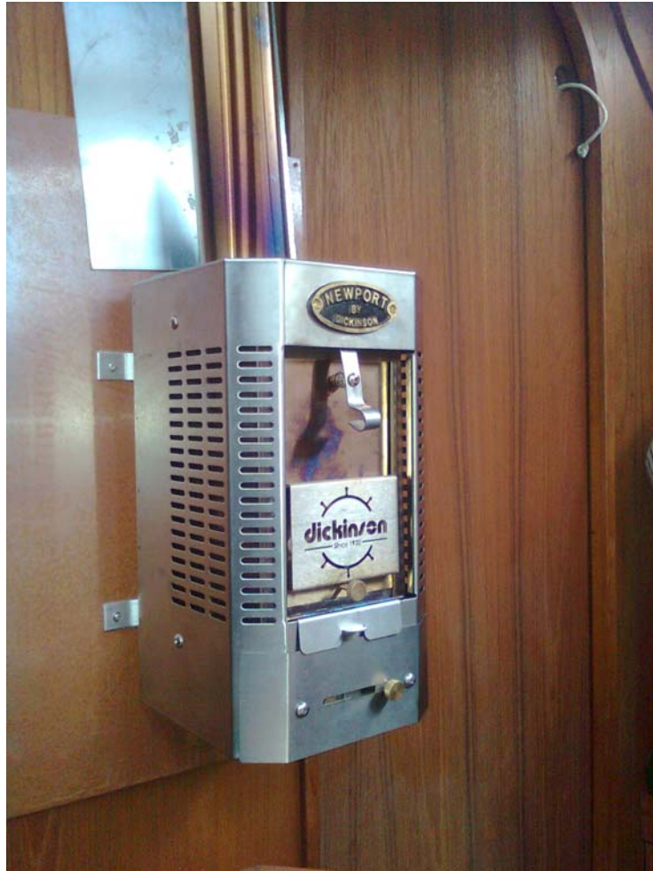
Dickinson Newport solid fuel heater, bolted onto the main bulkhead of ED
